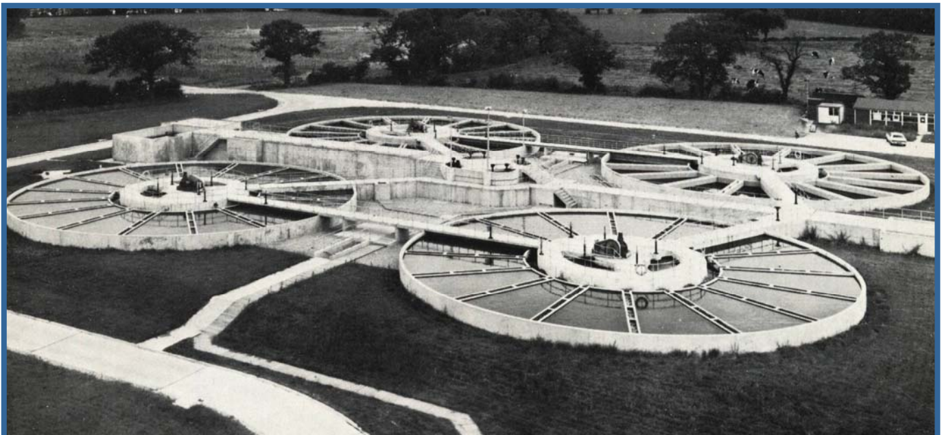
Typical installation of PCI Accentrifloc Clarifiers
